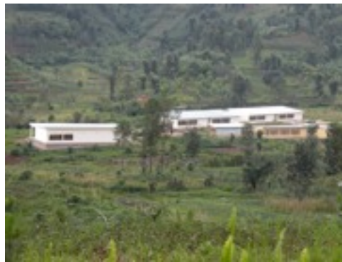
Kageno compound from afar, Banda Village
